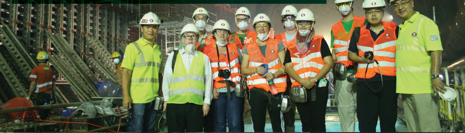
→ Some of the candidates and IOM 3 representatives at the MTR underground construction site.
