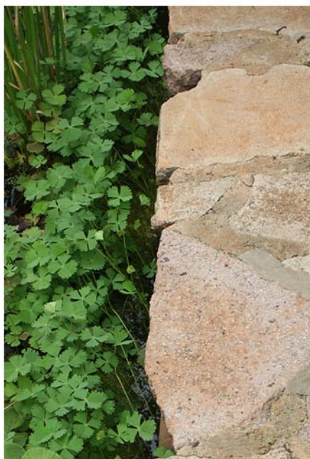
Retaining walls clad with recycled paving from previous walkways – the gaps inbetween provide habitat for reptiles and amphibians.
