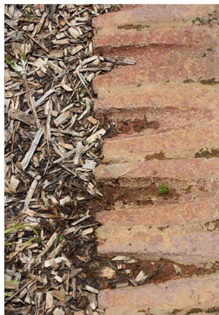
Grooved clay bricks that were previously used as wall cladding have been retained and used as edging for funneling stormwater into the planted landscape.
