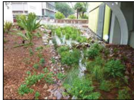
Vegetated swale entry point for surface storm water collection
