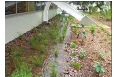
Vegetated swale (north side) collecting storm water from the roof and surrounding hard surfaces
