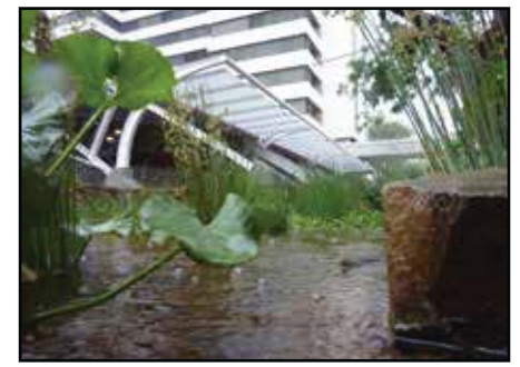
Tidal pond collecting storm water during a rain storm
