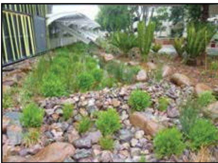
Vegetated swale entry point (north side) for surface storm water collection with Berula erecta and some of the cycads
