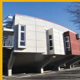
p 20 – Major infrastructure development completed
