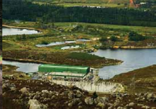
→ The Palmiet pump storage scheme in Grabouw.
