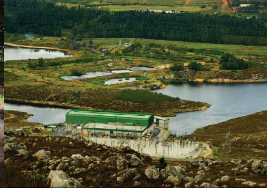
→ The Palmiet pump storage scheme in Grabouw.
