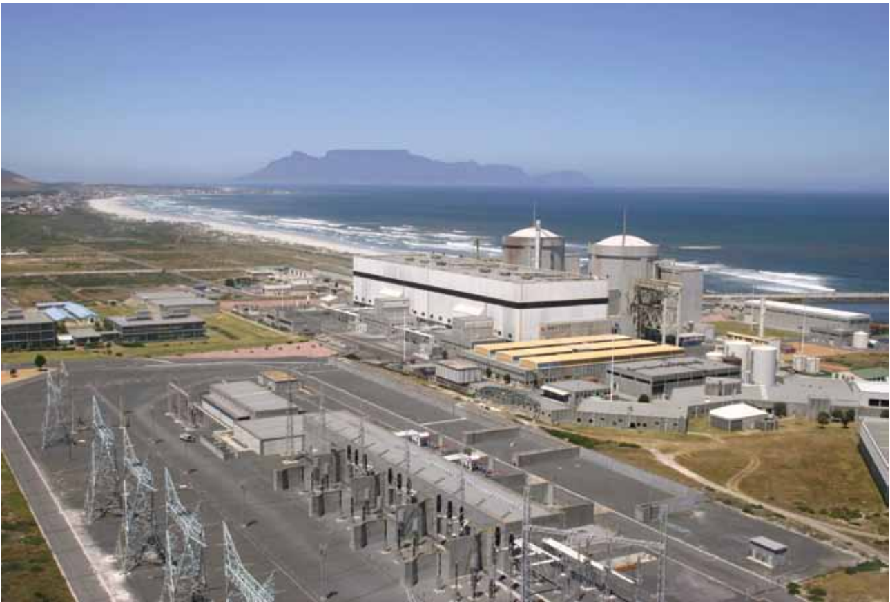
→ The Koeberg nuclear power plant.
