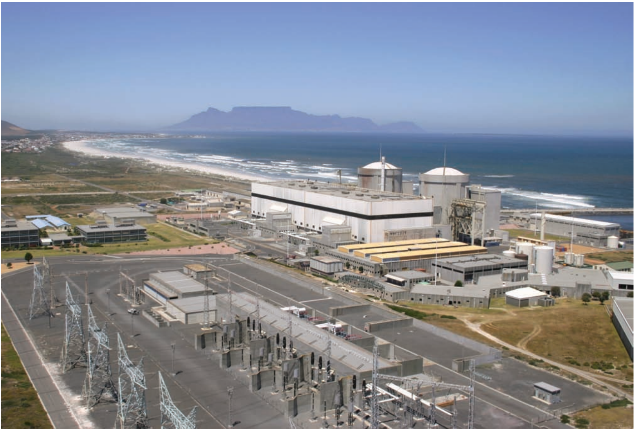
→ The Koeberg nuclear power plant.
