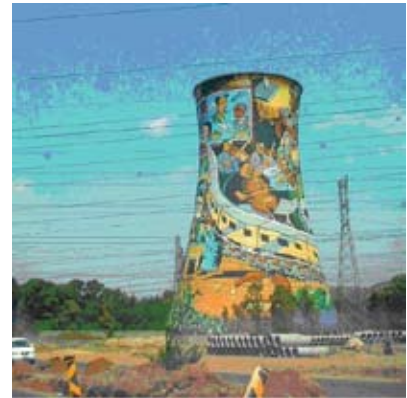
→ 5. Cooling-tower at Soweto power station: problem of risk-distribution.
