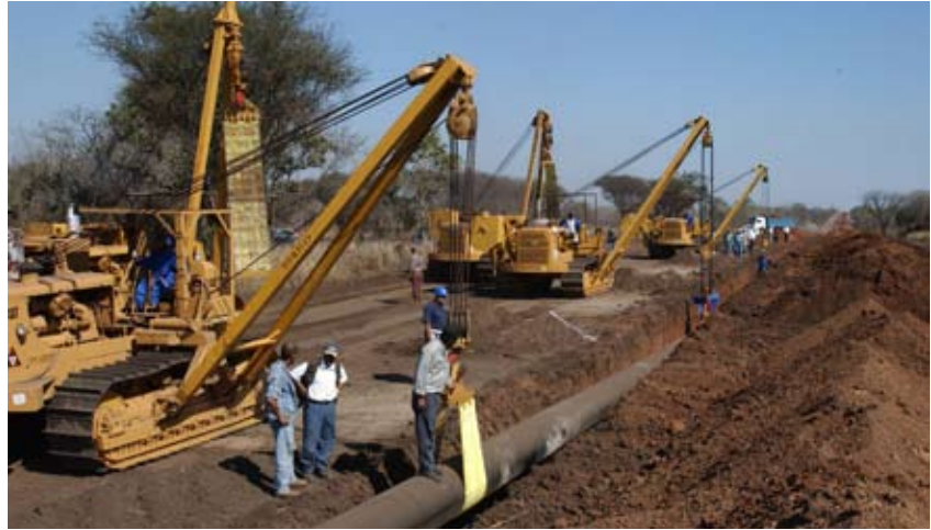
→ 1. Gas pipe laying from Mozambique to Secunda
