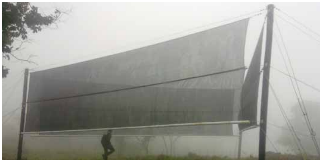
A newly operational triangular designed fog net, trapping fog at Tshanowa Primary School, March 2013. Picture: Prof Van Heerden.
